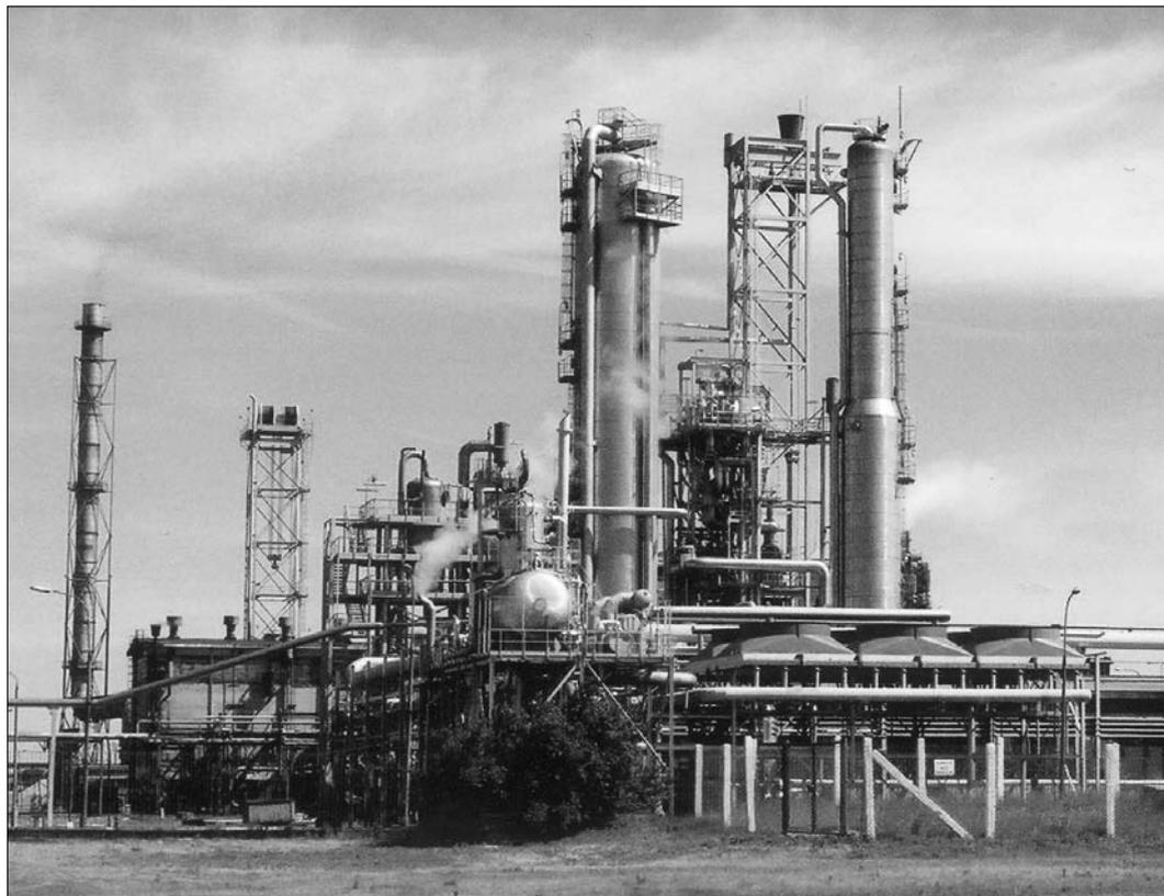
Chemical Fertiliser Plant) currently produces sulphuric acid, phosphoric acid, single and granulated superphosphate, di-ammonium phosphate and aluminium fluoride. Other large plants exist in Novgorod in Russia and Köping in Sweden.
